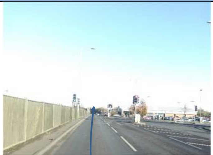
8.4.5.2. – View of splitter island
