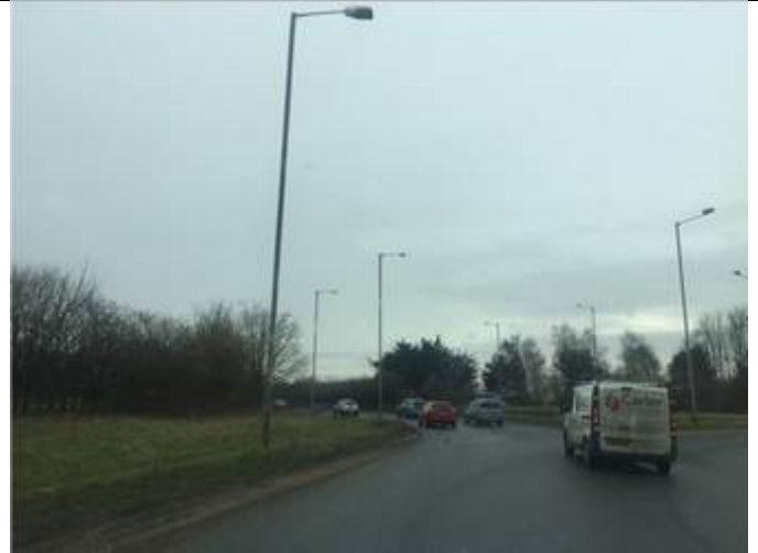
8.8.1.4. – View of exit of roundabout
