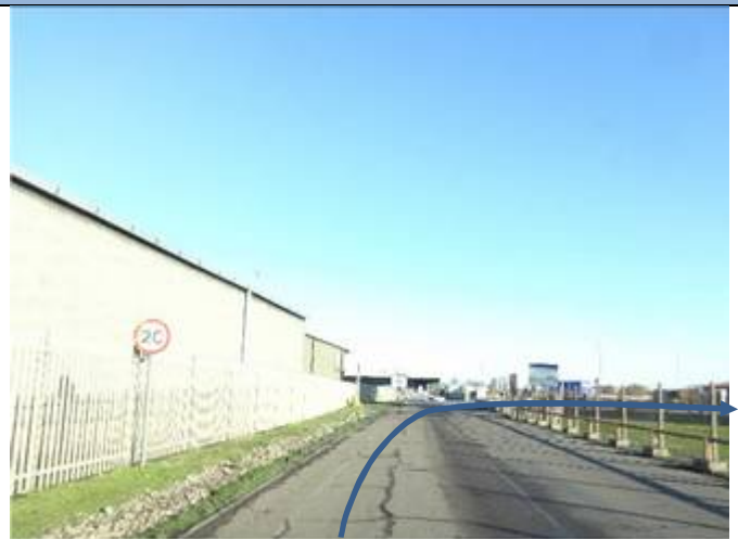
8.4.2.2. – View prior to bend
