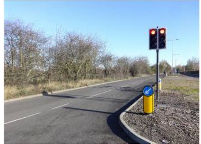
8.5.1.3. – View on junction
