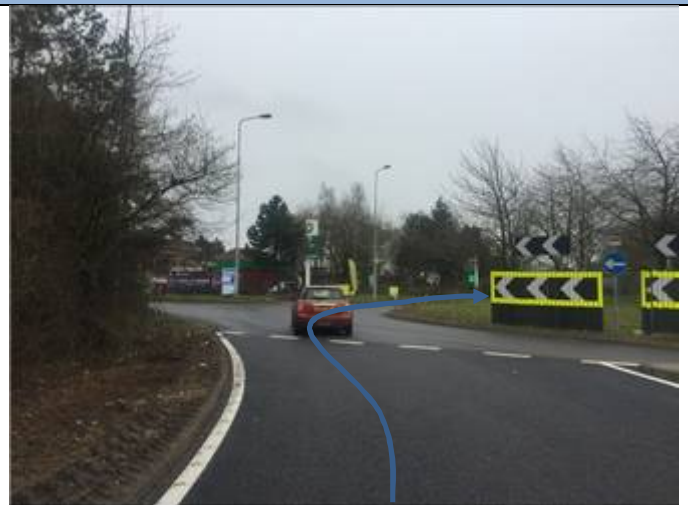
8.8.3.2. – View of entrance to roundabout
