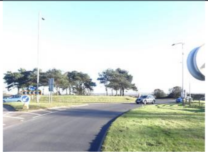
8.6.1.2. – View on prior to roundabout
