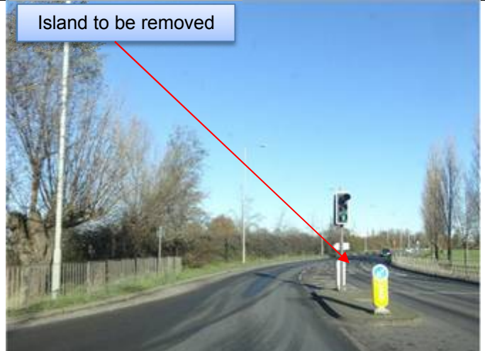
8.4.6.4. – View on junction
