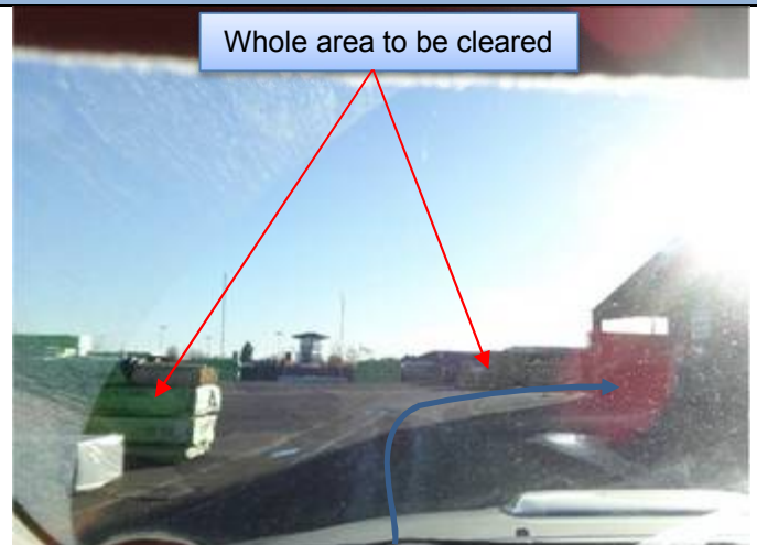
8.4.3.2. – View prior to bend
